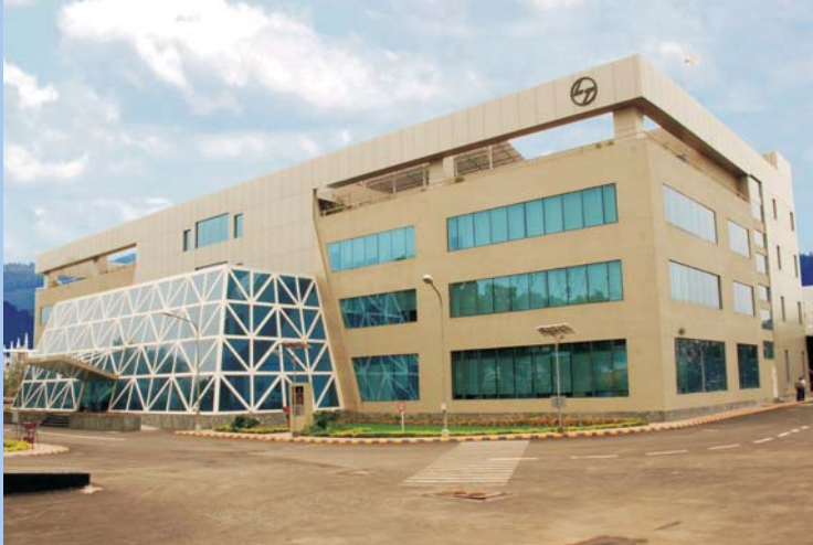
Switchgear Factory, Navi Mumbai
