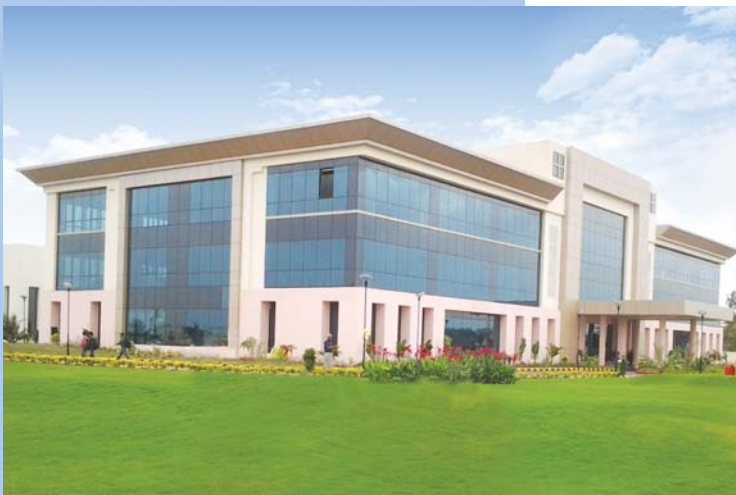
Switchgear Factory, Vadodara
