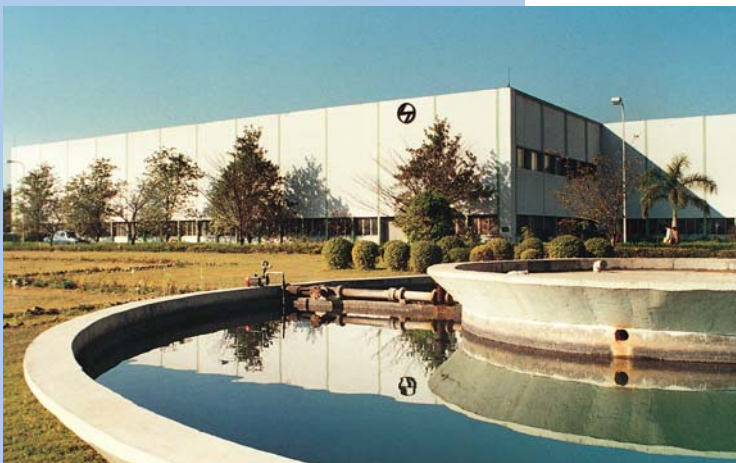
Switchgear Factory, Ahmednagar
